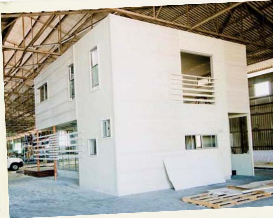
The first Smarter Small Home has been built in a hangar in QLD. It has achieved a 5.5 star rating, modelled with the BERS Pro 4.1 in Climate Zone 2.
